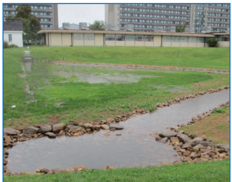
Stormwater Detention Basin Retrofits
