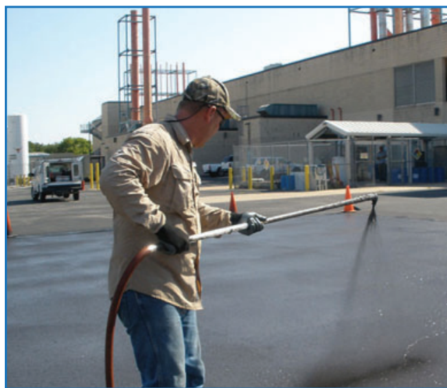
Stormwater runoff from coal-tar sealed parking lots is a major source of PAHs.
